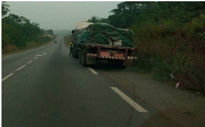
Figure 3. Parked vehicle by the roadside occupying part of the vehicle lane since shoulder width is insufficient
