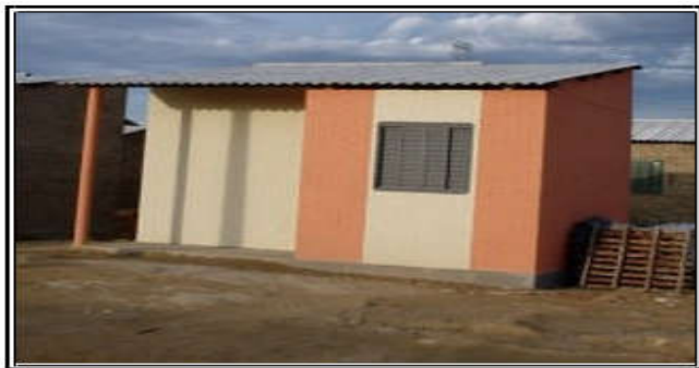
Figure 8. Soil-cement house ready to be delivered to the population
