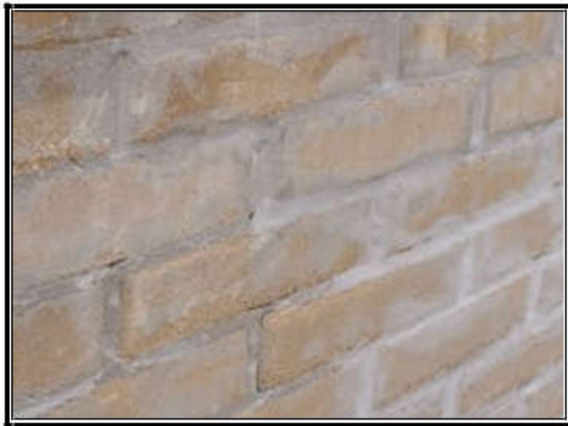
Figure 1. Grouted soil-cement wall.
