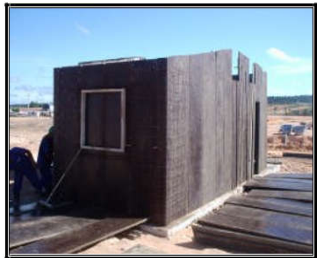
Figure 4. Partial lyre in for cedcellular concrete wall.
