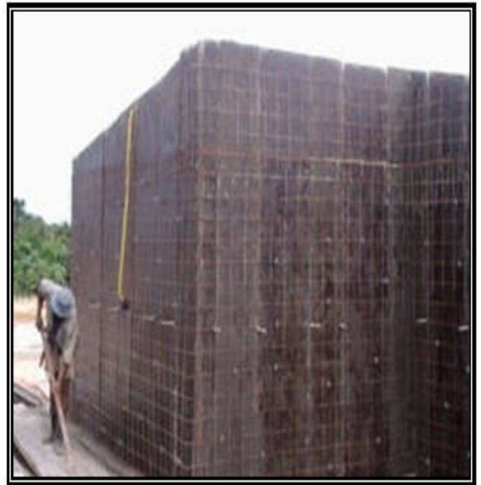
Figure 3. Reinforced cellular concrete wall.
