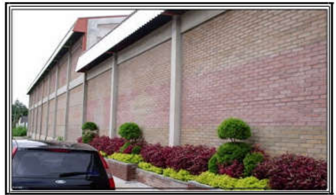
Figure 9. Industrial shed made of soil-cement bricks
