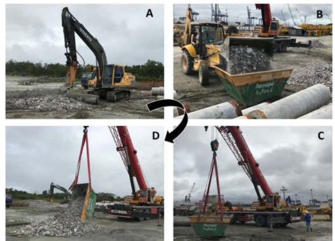
Figure 2. The sequence of activities of the second stage of investigation: A) breaks; B) load; C) weighing and D) discharge
