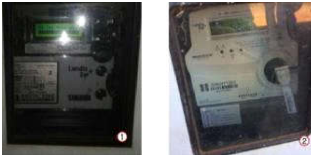
Figure 16. (1) Poultry house A1. Electronic energy meter Landis Gyr model Saga 1500 (2) Poultry house A2. Landis Gyr model E34A polyphase electronic meter
