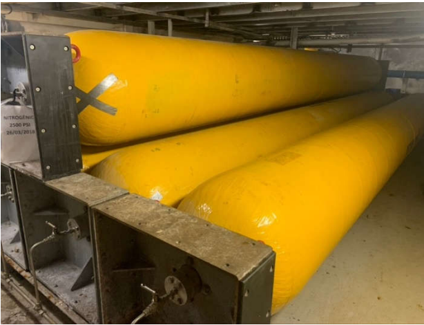
Fig. 1. CAPV's fabricated with Glass fiber epoxy and polyethylene high density
