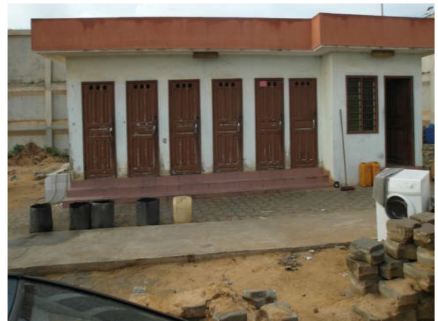
Figure 7. Picture showing a toilet cabins in the Port of Cotonou area
