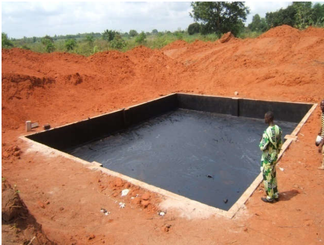
Figure 6. Tomb carried out for the destruction of the batteries (dangerous products)
