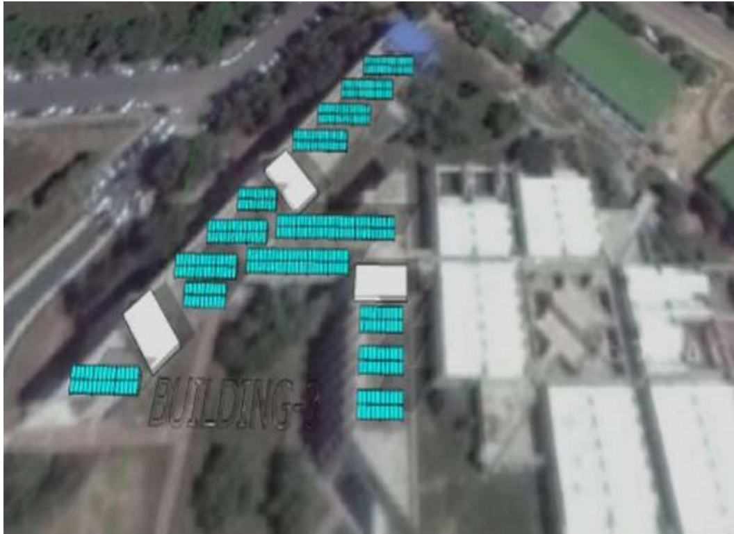
Figure 6.3: View of SPV installed at Building-3
