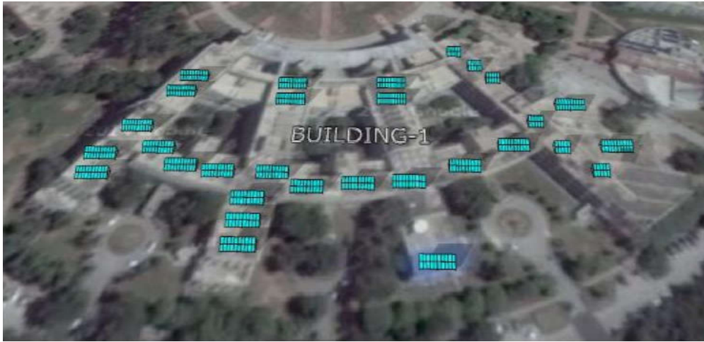
Figure 6.1- View of SPV installed at Building-1
